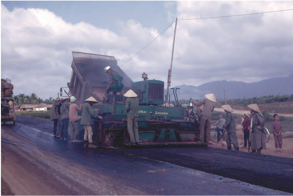
RMK-BRJ paves a portion of Highway 1 north of Qui Nhon.
